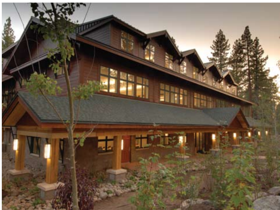
A Capstone C30 microturbine helps the Tahoe Center for Environmental Studies in California achieve LEED® certification.
