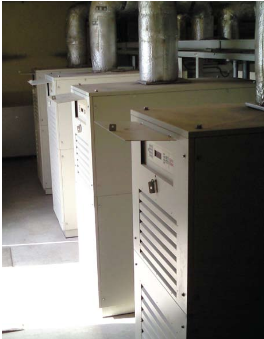
Methane gas fuels four C30 microturbines at a garbage-processing center in Japan.
