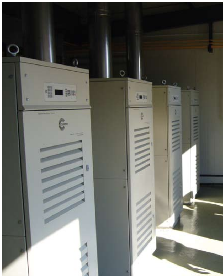
Five C60 microturbines provide electricity and heating for shopping malls, offices and warehouses in Yakutsk, Russia.
