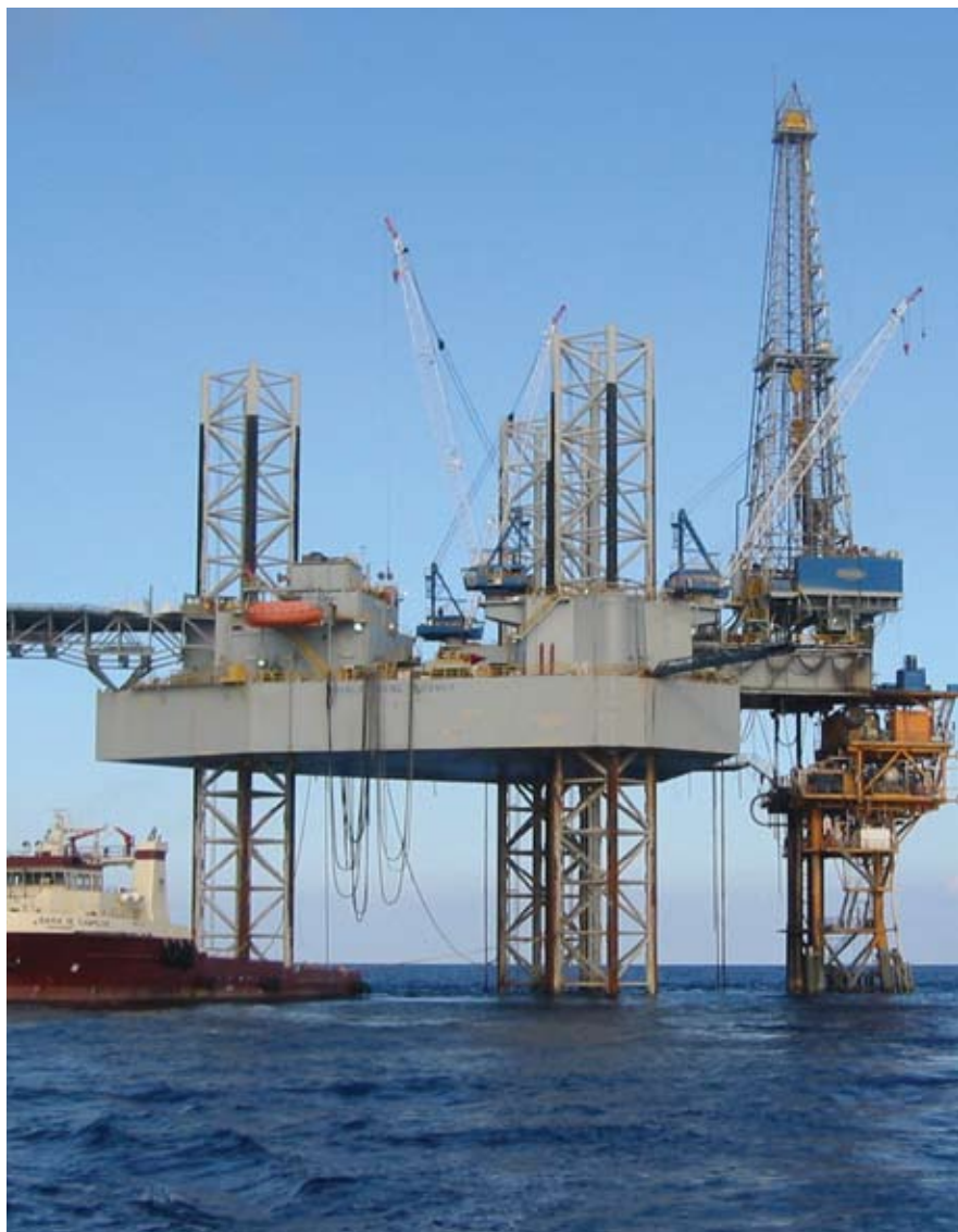
Two Capstone C30, class I, Division microturbines power this offshore platform in the Gulf of Mexico.
