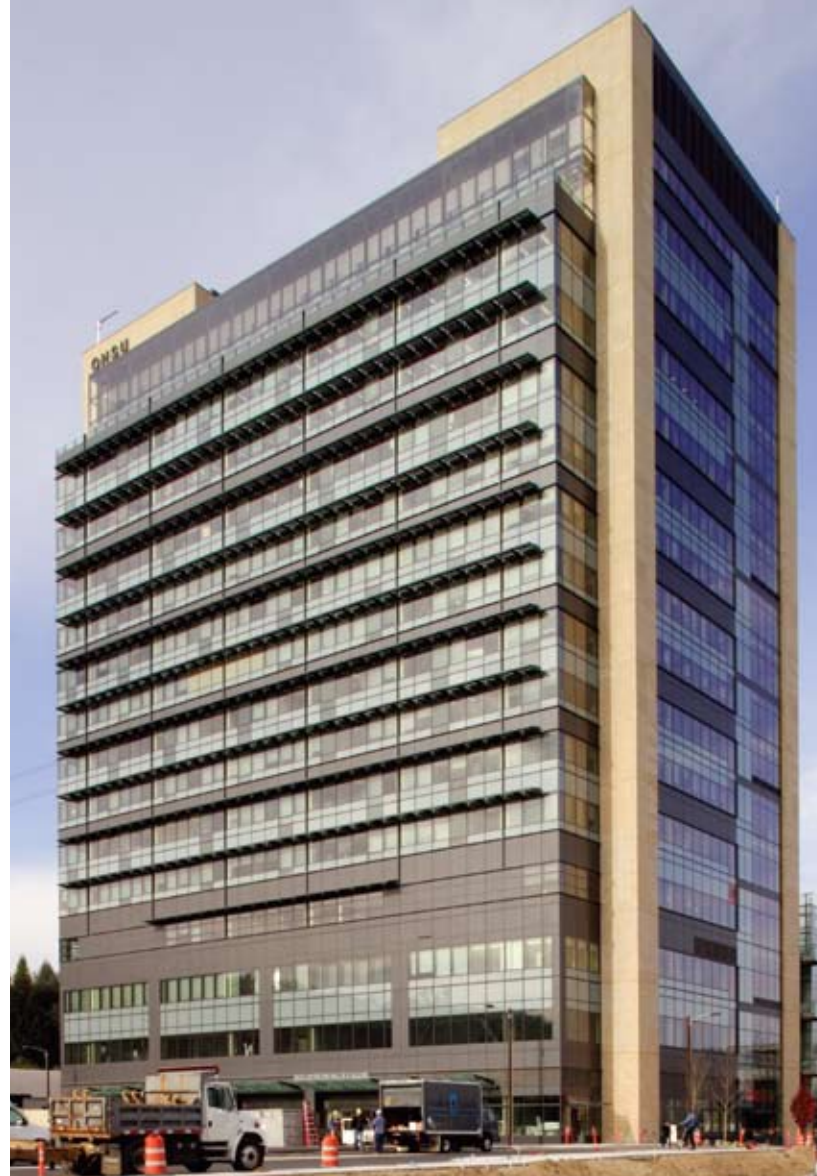
Five C60 ICHP microturbines used in a CHP application have reduced energy costs at this center for health and healing.
