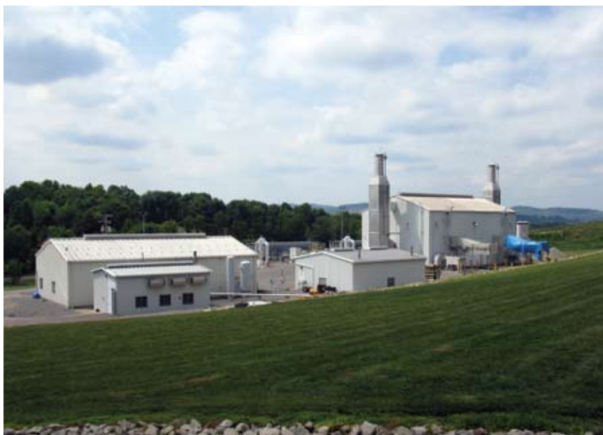
Dominion Transmission's Crayne Compressor Station in Pennsylvania, where three Capstone C65 ICHP microturbines provide all electricity and heat for the 5-acre site.
