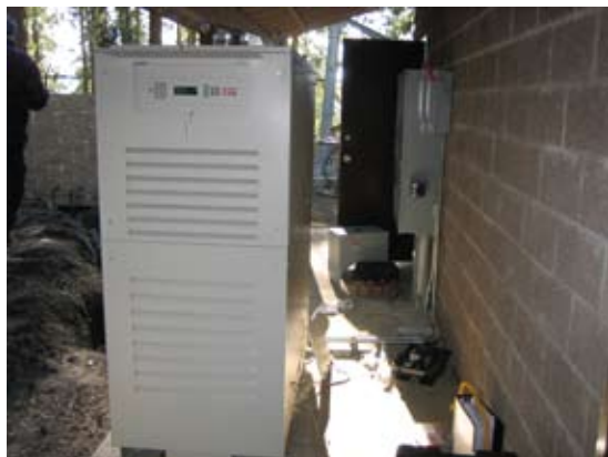
Four C65 MicroTurbines™ running on natural gas provide CCHP at a data center in California.
