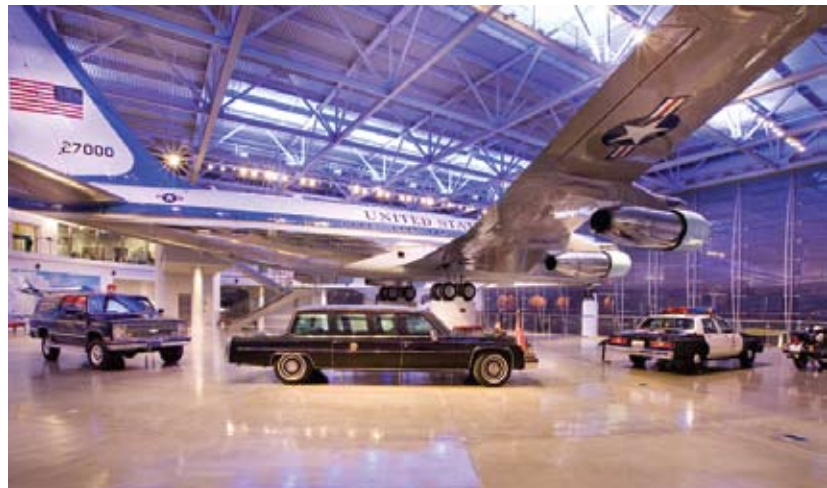
Sixteen Capstone C60 microturbines running on natural gas provide electricity for the Air Force One Pavillion.
