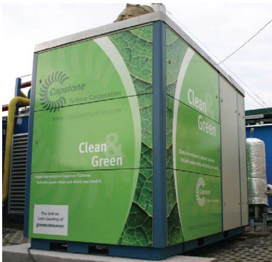
Capstone's CR200 microturbine provides up to 200 kW of power.
