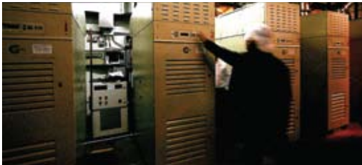
Capstone microturbines provide cooling, heating and power at Astor Chocolate in New Jersey.
