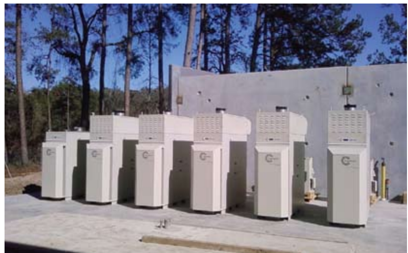
Six Capstone C65 microturbines generate continuous power at this U.S. government office.
