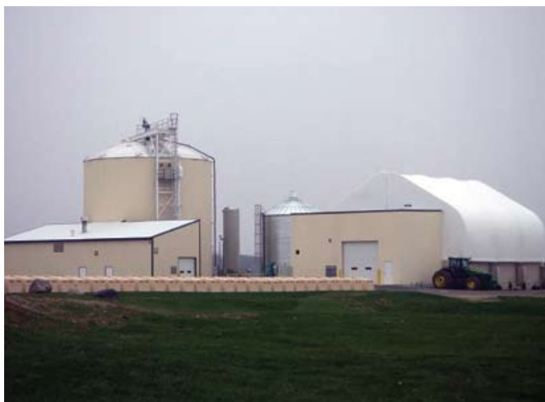
Waste methane gas from the 47 foot tall anaerobic digester fuels a Capstone microturbine that produces 30kW of clean, green electricity and 45kW of thermal energy used for building heat.
