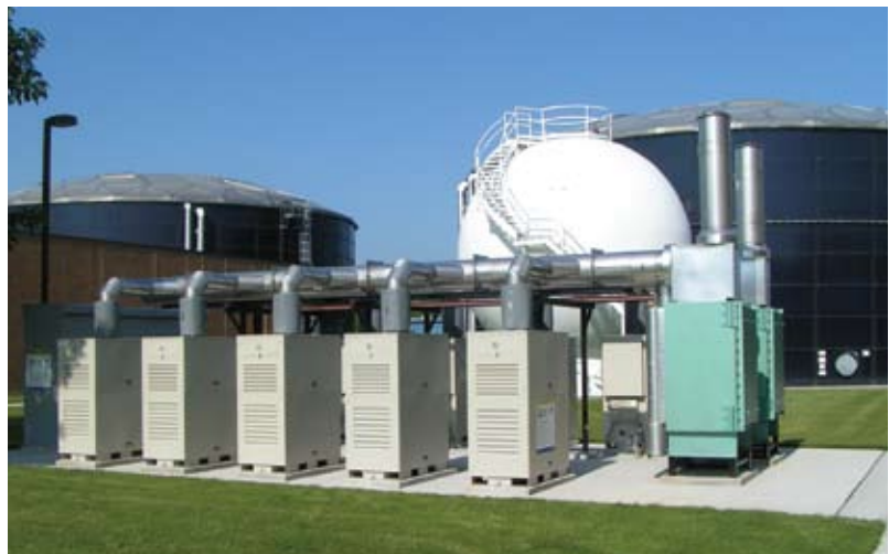
The Sheboygan Wastewater Treatment Plant has 10 low-emission Capstone microturbines that use methane gas created by solid waste to generate onsite electricity and heat, cutting the plants electric and natural gas bills by 40 percent and earning renewable energy and emissions credits.
